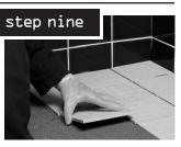
9. Allow membrane to dry for minimum 24 hours before tiling. When dry, background is suitable for BAL ready-mixed or cementitious powder adhesives. No priming required.
