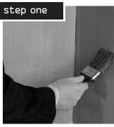
1. Prime all surfaces with **BAL PRIME APD** and allow to dry.
