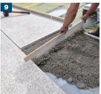
Using 50mm thick timber batons/rules on the AquaDrain® EK, apply the mixed drainage mortar in between the batons. Flatten until you reach the height of the timber battons. Once flattened, using a screeding bar, rule off to remove any excess mortar to provide a flat (50mm) bed. When used over 50mm, introduction of a reinforcing mesh should be considered.
