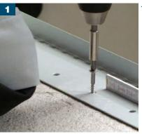
Prior to screw fixing the ProFin® DP and corner section, apply multi-purpose adhesive to the underside of the profile, minimum every 3 holes.
