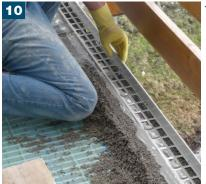
When not using ProFin® BL24/BL49, place the ProFin® V22 within the drainage screed to the height required to allow for a flush finish once the tile/stone is bedded using a BAL Flexible Tile Adhesive. ProFin® V22 should be used on an installation with a pre-existing roofing membrane and guttering system.
