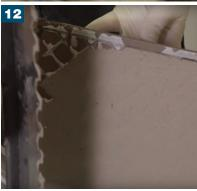
Apply a thin layer of adhesive over the whole back of the tile/stone using BAL RAPIDSET FLEXIBLE FIBRE adhesive. Apply a cone of adhesive using a 10mm notched trowel. A rubber mallet can be used to bed the tiles into the MorTec® DRAIN whilst still wet.
