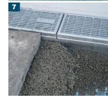
Place the plastic AquaDrain® Lochwinkel Screed Angle profile 70/50 where the AquaDrain® FLEX will meet the drainage mortar.
