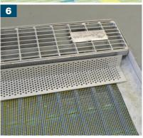
Place the powder coated steel AquaDrain® Lochwinkel Screed Angle profile 30/40 where the AquaDrain® TM will meet the drainage mortar.
