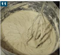
Once the MorTec® DRAIN drainage screed has been laid, mix up BAL RAPIDSET FLEXIBLE FIBRE. Refer to BAL TECHNICAL DATE SHEET on mixing.
