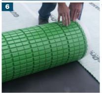
■ Loose lay PE Foil or plastic sheeting (0.2mm thick) on to floor to give extra protection. Roll out the AquaDrain® T+ matting and cut to size using inclustrial scissors or utility knife. Ensure that the waterproofing is not cut.
