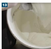
Once the adhesive is dry after 3 hours, clean down the surface and leave to dry before mixing the cement based grout such as BAL MICROMAX2 grout. Refer to BAL TECHNICAL DATE SHEET for information on mixing and application.
