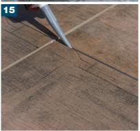
Once the grout is dry after a minimum of 3 hours, a silicone sealant such as BAL MICROMAX SEALANT or MorTec® SOFT can be used to apply a soft bead of sealant around the perimeter edge, movement joints, and where the tile/stone meets the AquaDrain® TM and edge profiles i.e. ProFin® BL24/ BL49 or ProFin® V22 and at intermediate movement joints at 3m intervals maximum. Refer to **BAL TECHNICAL DATA SHEET** for further information.
