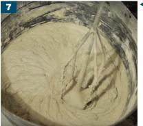
Mix up BAL STONE & TILE PTB tile adhesive. Refer to BAL TECHNICAL DATA SHEET on mixing.
