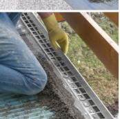
When not using ProFin® DP21 and ProFin® BL49, place the ProFin® V55 within the drainage mortar to the height required to allow for a flush finish once the tile/stone is bedded using a BAL Flexible Tile Adhesive. ProFin® V55 should be used where roof membrane and gutter system is pre-installed.
