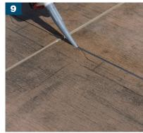
Once the adhesive is set, gun apply MorTec® SOFT sealant to the open joints of the tiles, around the perimeter edge, on intermediate movement joints and where the tile/ stone meets the AquaDrain® TM drain grate and edge profiles i.e. ProFin® BL24 DP11 and ProFin® DP30. Refer to BAL TECHNICAL DATA SHEET on application.
