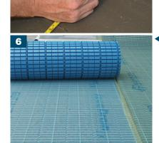
■ Roll out the AquaDrain® EK matting and cut to size using industrial scissors. Ensure that the waterproofing is not cut.
