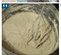
Once the drainage mortar has been laid, mix the BAL RAPIDSET FLEXIBLE FIBRE as per the relevant BAL TECHNICAL DATA SHEET.
