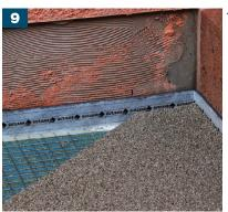
■ Using 25mm thick timber batons/rules placed on the AquaDrain® EK sheets, apply the mixed MorTec® DRAIN epoxy drainage screed in between and flatten until you reach the height of the timber batons. Flatten using a screeding bar, rule off to remove any excess mortar to provide a flat (25mm) bed of drainage screed.
