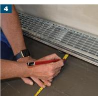
It's always good practice to measure and mark the depth of the AquaDrain® TM drain before laying the PE Foil and rolling out the AquaDrain® T+ drainage mat.
