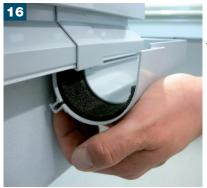
Once completed attach the ProRin® BR guttering system to ProFin® DP11 or ProFin® DP21 edge profile.
