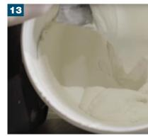
Once the adhesive is dry after 3 hours, clean down the surface and leave to dry before mixing a cement based grout such as BAL MICROMAX2 grout. Refer to BAL TECHNICAL DATA SHEET for information on mixing and application.
