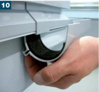
◆ Once completed attach ProRin® BR drainage guttering to ProFin® DP11/ DP21 or ProFin® DP30 if required. See ProRin® BR BAL TECHNICAL DATA SHEET for full installation instructions.
