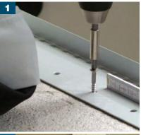
Prior to screw fixing the ProFin® DP and corner section, apply multi-purpose adhesive to the underside of the profile, minimum every 3 holes. Screw fix ProFin® DP11 or ProFin® DP30 edge profile into position onto the existing base. External corners (90°) ProFin® DP11/ProFin® DP21 or ProFin® DP30 and profile connectors are available. Use the screws and rawlplugs provided and fix screws at either end of profile and every 500mm.
