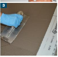
Apply BAL TANK-IT tape to the overlaps then apply two coats of BAL TANK-IT onto the bonded, sloped screed and up to the plastic side of the DiProtec® AB-KV sealing tape, covering the fleece. Please refer to BAL TECHNICAL DATA SHEET for application information. Allow 30mins drying time before applying a second coat
