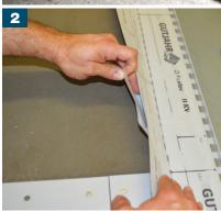
▼ Following installation of the DP profile, use the self-adhesive DiProtec® AB-KV sealing tape as a seal between the profile and the substrate. Fix the plastic side to the edge profile (do not cover drainage holes) and the fleece side to the bonded screed and flatten down with a roller.
