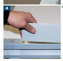
◀ Clip on the BL49 corner section and facing plates to the DP profile, leaving 5mm gap. Clip on connectors to bridge the gap, use multi-purpose adhesive for extra purchase. Loose lay PE Foil or plastic sheeting (0.2mm thick).
