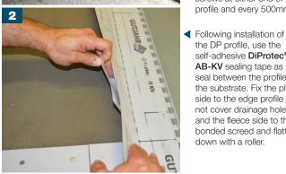
not cover drainage holes) and the fleece side to the bonded screed and flatten down with a roller. ■ Apply BAL TANK-IT tape to the overlaps then apply two coats of BAL TANK-IT onto the bonded, sloped screed and up to the plastic side of the DiProtec® AB-KV
