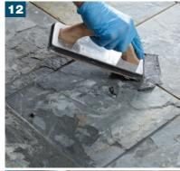
Apply BAL MICROMAX2 grout to the face of the tile and compact into each of the joints.
