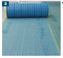
Using 50mm thick timber batons/rules on the AquaDrain® EK, apply the mixed drainage mortar in between the batons. Flatten until you reach the height of the timber batons. Once flattened, using a screeding bar, rule off to remove any excess mortar to provide a flat (50mm) bed of drainage mortar. When used over 50mm, introduction of a reinforcing mesh should be considered.
