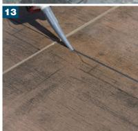
■ Once the grout is dry after a minimum of 3 hours, a silicone sealant such as BAL MICROMAX SEALANT or MorTec® SOFT can be used to apply a soft bead of sealant around the perimeter edge and where the tile/stone meets the AquaDrain® TM and edge profiles i.e. ProFin® V22. Sealant should also be applied to intermediate movement joints at 3m intervals Refer to BAL TECHNICAL DATA SHEET for further information.
