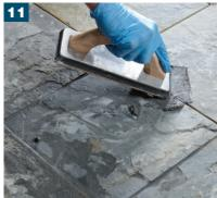
Apply the BAL MICROMAX2 and compact into each of the joints.
