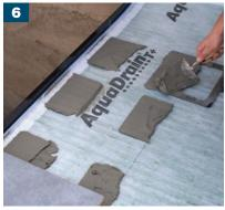
■ Before laying the 20mm porcelain tiles or the 30mm natural stone. Apply pads of adhesive (minimum 4mm thick) at a distance not exceeding 200mm, ensuring all four corners of the tiles are fully supported. Minimum tile dimensions 300mm x 300mm.
