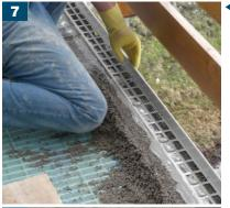
◆ Place the ProFin® V55 within the drainage mortar to the height required to allow for a flush finish once the tile/stone is bedded in adhesive.
