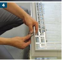
■ Lay the ProFin® V22 edge profile into position on top of the AquaDrain® T+ (Corner 90° and profile connectors are available.
