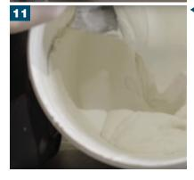
Once the adhesive is dry after 3 hours, clean down the surface and leave to dry before mixing the cement based grout such as BAL MICROMAX2 grout. Refer to BAL TECHNICAL DATA SHEET for information on mixing and application.
