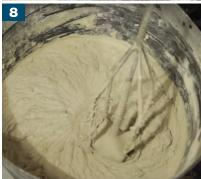
Once the drainage mortar has been laid, mix up BAL STONE & TILE PTB as per the relevant BAL TECHNICAL DATA SHEET.
