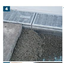
◆ Place the plastic AquaDrain® Lochwinkel Screed Angle profile 70/50 where the AquaDrain® FLEX will meet the drainage mortar.
