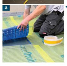
Place the AquaDrain® EK 8mm sheets down and cut to size using industrial scissors. Ensure that the waterproofing layer is not cut or damaged.
