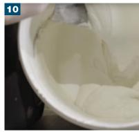
Once the adhesive is dry after 3 hours, clean down the surface and leave to dry before mixing cement based grout such as BAL MICROMAX2. Refer to BAL TECHNICAL DATA SHEET for information on mixing and application.
