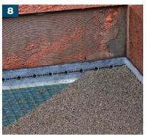
Using 25mm thick timber batons/rules placed on the AquaDrain® EK sheets, apply the mixed MorTec® DRAIN epoxy drainage screed in between and flatten until you reach the height of the timber batons. Flatten, using a screeding bar, rule off to remove any excess mortar to provide a flat (25mm) bed of drainage screed.
