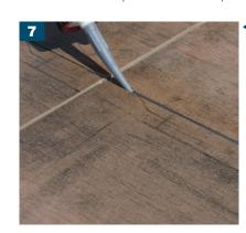
Once the adhesive is set, gun apply MorTec® SOFT sealant to the open joints of the tiles around the perimeter edge, movement joints, and where the tile/stone meets the AquaDrain® TM drain grate and edge profiles i.e. ProFin® V22. Also use to fill intermediate joints placed at 3m intervals. Refer to BAL TECHNICAL DATA SHEET on application.
