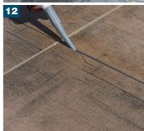
■ Once the grout is dry after a minimum of 3 hours, BAL MICROMAX SEALANT or MorTec® SOFT can be used to apply a soft bead of sealant around the perimeter edge, intermediate joints at 3m intervals and where the tile/stone meets the AquaDrain® FLEX and edge profiles i.e. ProFin® V55. Refer to BAL TECHNICAL DATA SHEET for further
