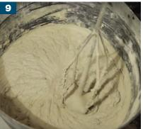
Once the MorTec® DRAIN has been laid, mix up BAL RAPIDSET FLEXIBLE FIBRE. Refer to BAL TECHNICAL DATA SHEET on mixing.
