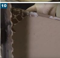
Apply a thin layer of adhesive over the whole back of the tile/stone using BAL RAPIDSET FLEXIBLE FIBRE adhesive. Apply a cone of adhesive to the back of the tile using a 10mm notched trowel. A rubber mallet can be used to bed the tiles into the MorTec® DRAIN, whilst still wet.
