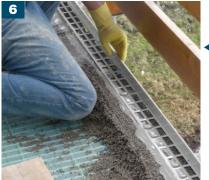
■ When not using the ProFin® BL24/BL49, place the ProFin® V22/V55 within the drainage screed to the height required to allow for a flush finish once the tile/stone is bedded using a BAL Flexible Tile Adhesive.
