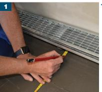
▼ Following the installation of ProFin® DP11/ DP21 and roofing grade membrane, loose lay PE Foil or plastic sheeting (0.2mm thick) onto the primary waterproofing layer. Measure and mark the depth of the AquaDrain® TM drain before laying the PE Foil and the AquaDrain® EK drainage sheets.
