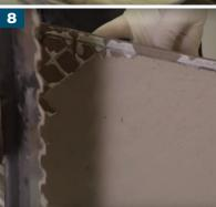
Apply a thin layer of adhesive over the whole back of the tile/stone using BAL RAPIDSET FLEXIBLE FIBRE adhesive. Apply a cone of adhesive using a 10mm notched trowel. A rubber mallet can be used to bed the tiles into the drainage screed, whilst still wet.
