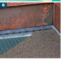
■ Using 25mm thick timber batton/rules placed on-to the AquaDrain® EK sheets, apply the mixed MorTec® DRAIN epoxy drainage screed in between and flatten until you reach the height of the timber battons. Flatten, using a screeding bar, rule off to remove any excess mortar to provide a flat (25mm) bed of drainage screed.
