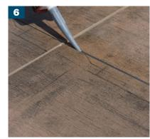
Once the adhesive is set, gun apply MorTec® SOFT sealant to the open joints of the tiles, around the perimeter edge, on intermediate movement joints and where the tile/ stone meets the AquaDrain® TM drain grate and edge profiles i.e. ProFin® BL24 / DP11 and ProFin® DP30 edge profiles. Refer to BAL TECHNICAL DATA SHEET on application.
