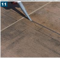
■ Once the grout is dry after a minimum of 3 hours, BAL MICROMAX SEALANT or MorTec® SOFT can be used to apply a soft bead of sealant around the perimeter edge, movement joints, and where the tile/stone meets the AquaDrain® FLEX and ProFin® V55. Intermediate movement joints should be placed at a maximum of 3m intervals. Refer to BAL TECHNICAL DATA SHEET for further information.
