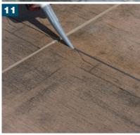
Once the grout is dry after a minimum of 3 hours, a silicone sealant such as BAL MICROMAX SEALANT or MorTec® SOFT can be used to apply a soft bead of sealant around the perimeter edge, movement joints, and where the tile/stone meets the AquaDrain® TM and edge profiles i.e. ProFin® BL24/ **BL49**. Intermediate movement joints should be placed at a maximum of 3m intervals. Refer to BAL TECHNICAL DATA **SHEET** for further information.
