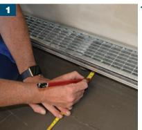
▼ Following the installation of the waterproof membrane and ProFin® DP11 or DP30, loose lay PE Foil or plastic sheeting (0.2mm thick) on to floor to give extra protection, measure and mark the depth of the AquaDrain® TM drain grate before laying the PE Foil and rolling out the AquaDrain® T+ drainage mat.
