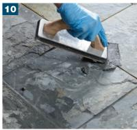
Apply the BAL MICROMAX2 and compact into each of the joints.
