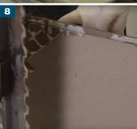
Apply a thin layer of adhesive over the whole back of the tile/stone using an adhesive such as BAL RAPIDSET FLEXIBLE FIBRE adhesive. Apply a cone of adhesive using a 10mm notched trowel. A rubber mallet can be used to bed the tiles into the drainage mortar whilst still wet.
