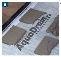
■ Before laying the 20mm porcelain tiles or the 30mm natural stone, Apply pads of adhesive (minimum 4mm thick) at a distance not exceeding 200mm, ensuring all four corners of the tiles are fully supported.
