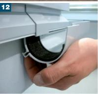
Once completed attach the ProRin® BR guttering system to ProFin® DP11 or ProFin® DP21 edge profile. See ProRin® BR BAL TECHNICAL DATA SHEET for full installation instructions.
