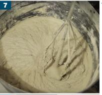
Once the drainage mortar has been laid, mix up BAL RAPIDSET FLEXIBLE FIBRE as per the relevant BAL TECHNICAL DATA SHEET.
