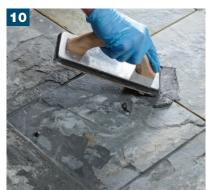
Apply BAL MICROMAX2 grout to the face of the tile and compact into each of the joints.
