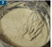
Once the MorTec® DRAIN has been laid, mix up BAL RAPIDSET FLEXIBLE FIBRE tile adhesive. Refer to BAL TECHNICAL DATA SHEET on mixing.
