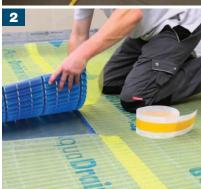
Place the AquaDrain® EK 8mm sheets down and cut to size using industrial scissors. Ensure that the waterproofing is not cut.
