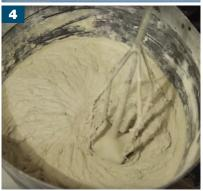
Mix up BAL STONE & TILE PTB tile adhesive. Refer to BAL TECHNICAL DATA SHEET on mixing.
