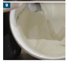
Once the adhesive is dry after 3 hours, clean down the surface and leave to dry before mixing the cement based grout such as BAL MICROMAX2 grout. Refer to BAL TECHNICAL DATA SHEET for information on mixing and application.
