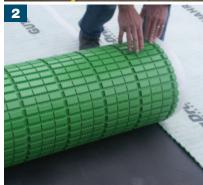
Roll out the AquaDrain® T+ matting and cut to size using industrial scissors. Ensure that the waterproofing is not cut.
