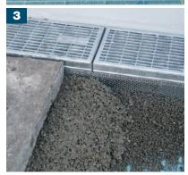
◆ Place the plastic AquaDrain® Lochwinkel Screed Angle profile 70/50 where the AquaDrain® FLEX drain grate will meet the drainage mortar
